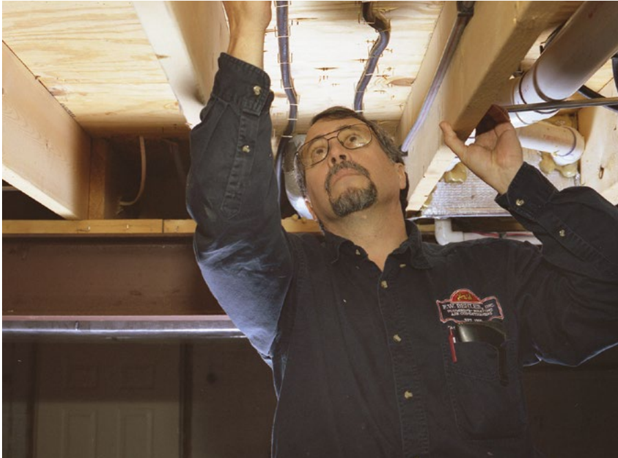
Dave Yates checks installed Onix tube staple-up. Photo by John Herr.
