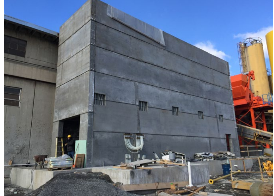
The radiant bunker completed.
