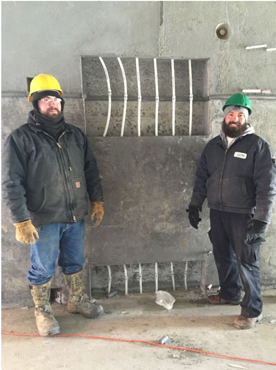
Bitter cold weather was an ongoing challenge on this project.
