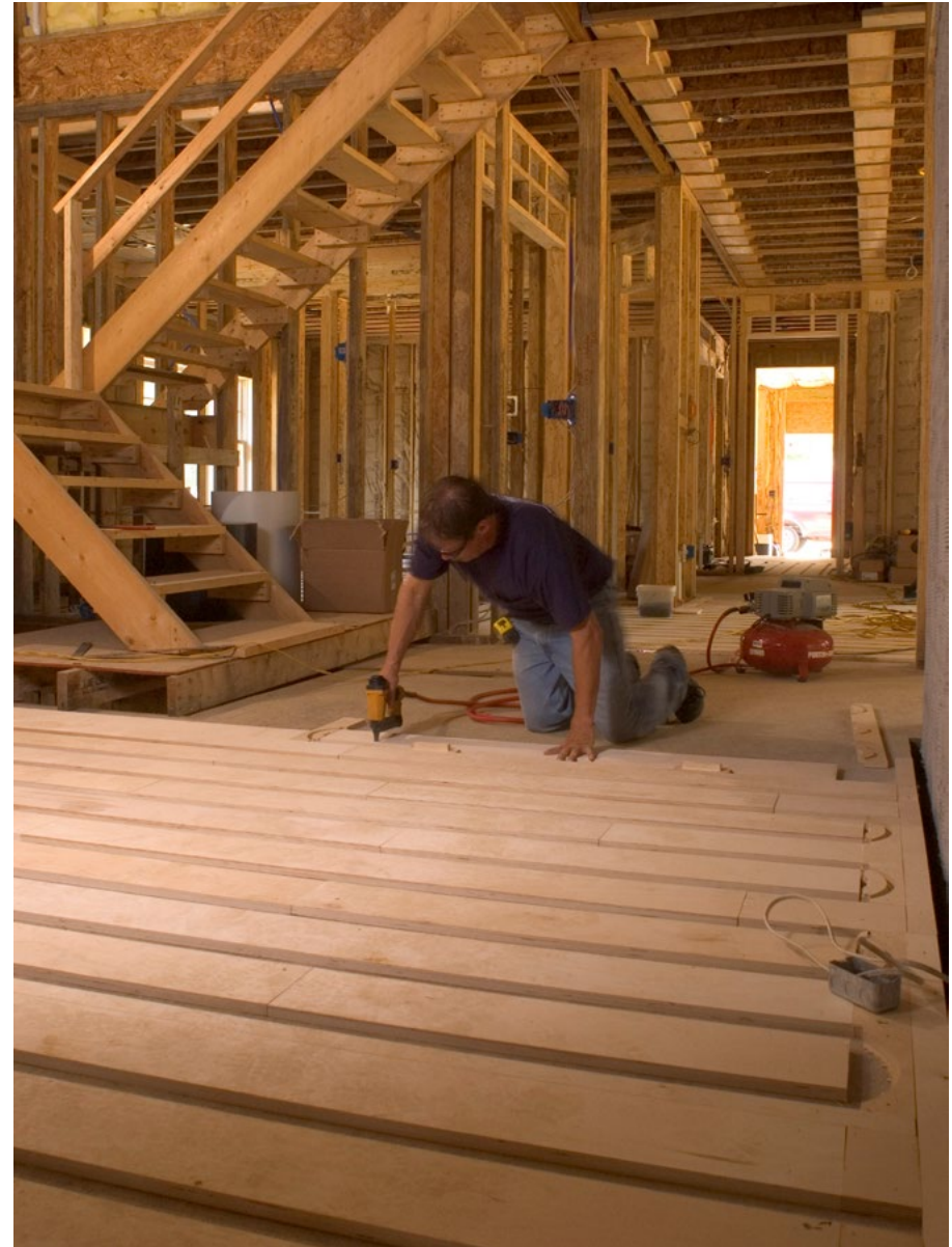
A Behler technician installs Watts SubRay panels.
