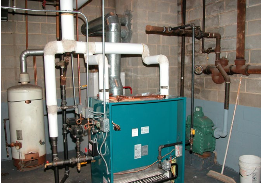
The new steam boiler in place.
