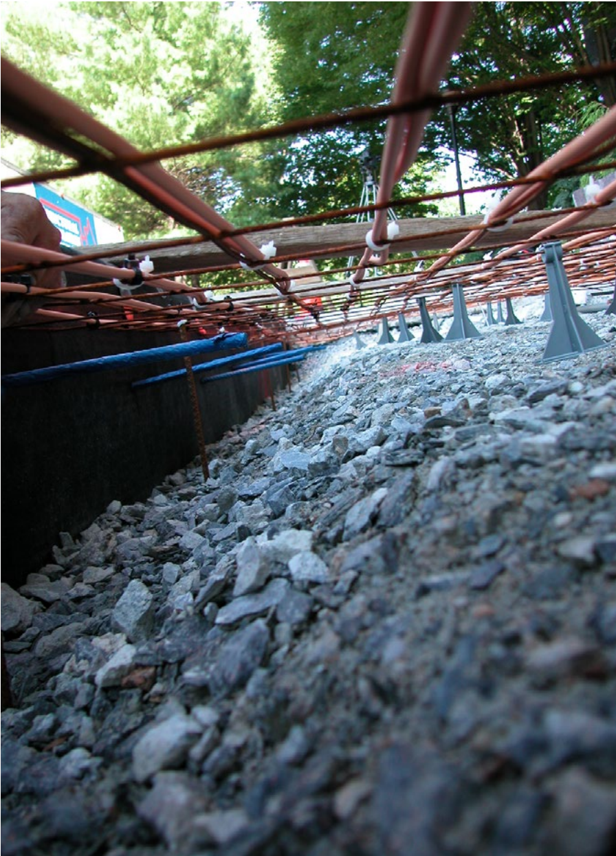
A view of the underside wire grid supported by chairs.
