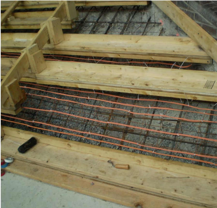
The stairway cables are installed.
