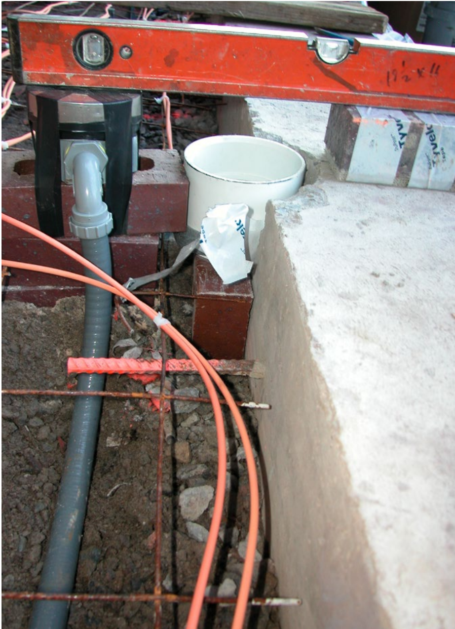
A Watts snow melt sensor body is installed.
