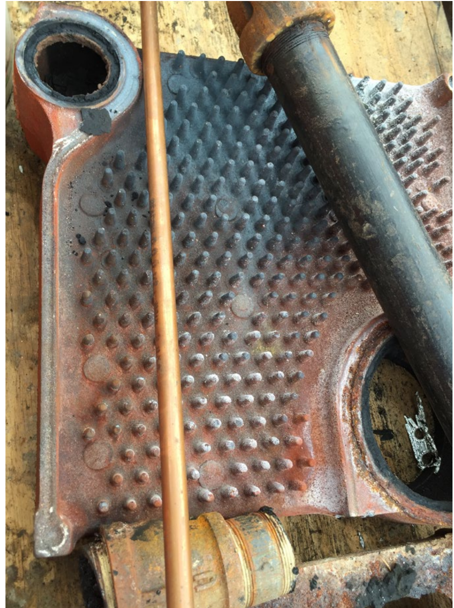
Cracked cast iron sections of a neglected steam boiler.
