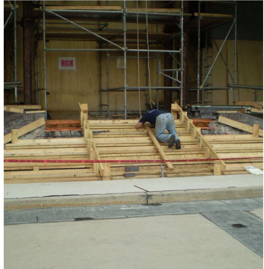
The stairway cables installation.
