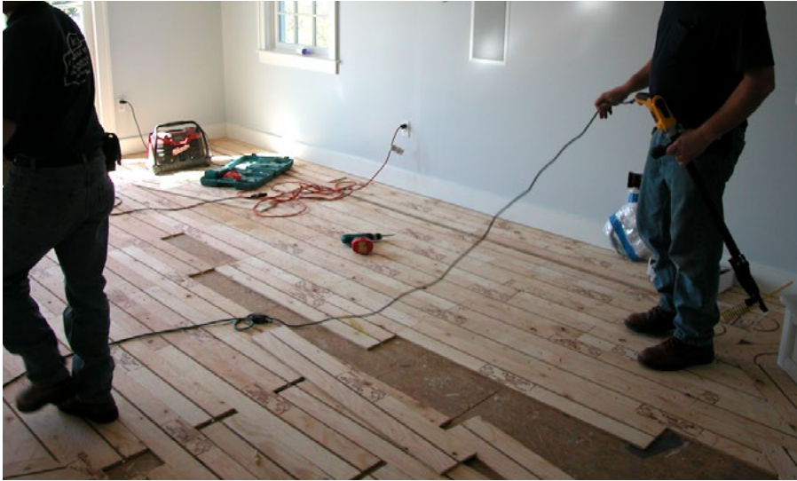
Installing QuikTrack in the master bedroom.
