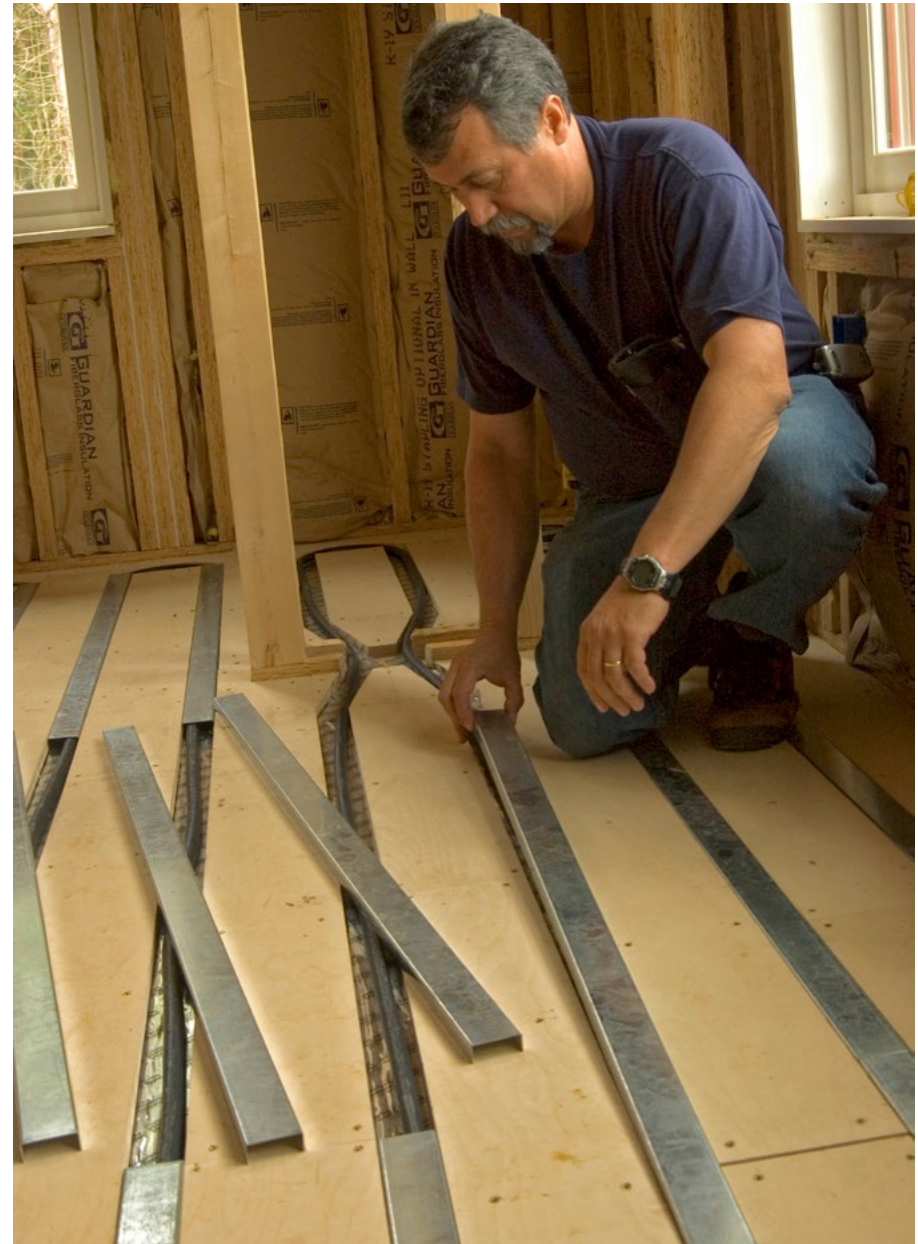
Dave Yates installs metal plates over Onix tubing in SubRay panels.
