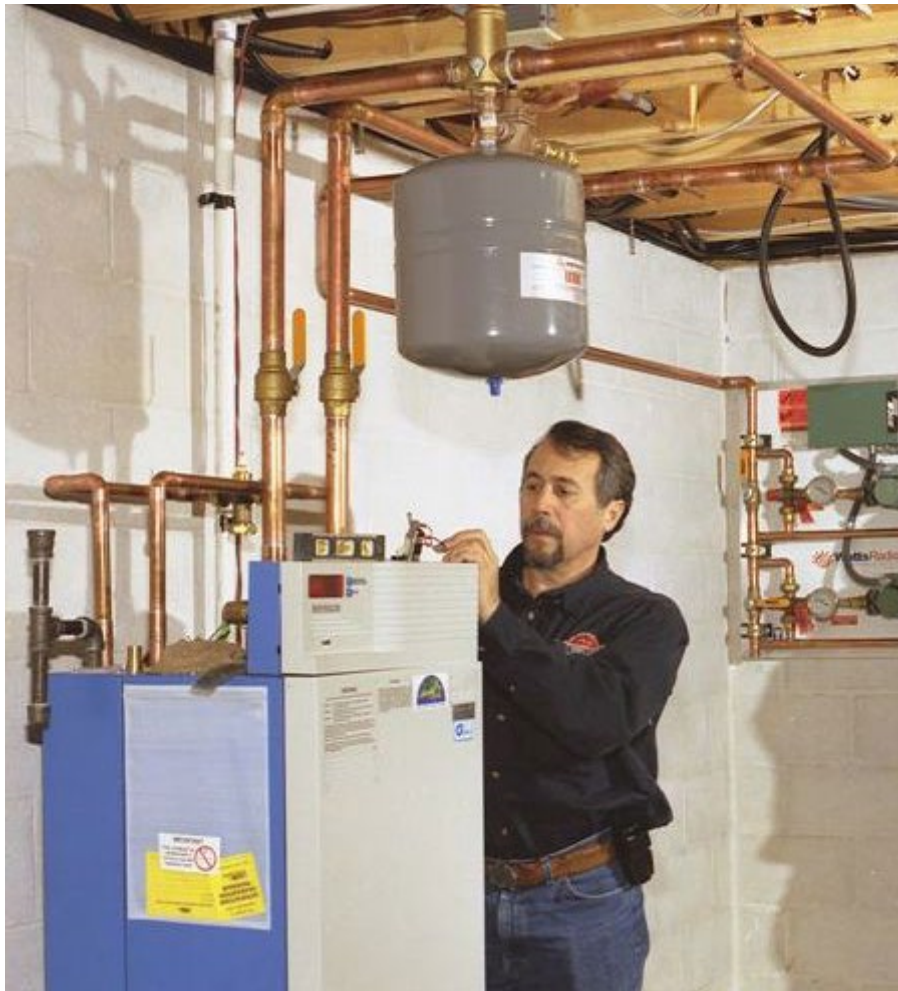
Dave Yates completes wiring for Laars boiler. Photo by John Herr.
