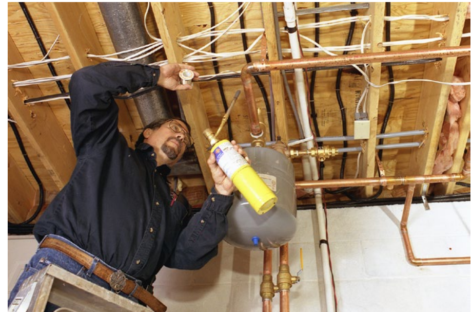
Dave Yates solders hydronic piping. Photo by John Herr.
