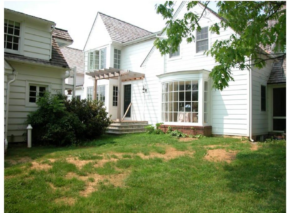
The final combined combustion exhaust/intake, located away from the home.
