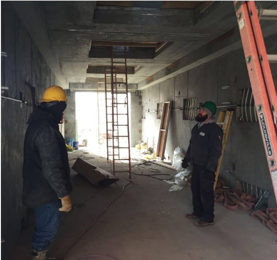
The lower floor of the radiant bunker.
