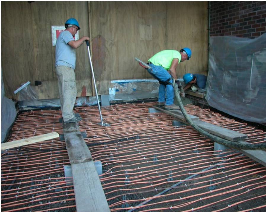
The concrete pour getting underway.
