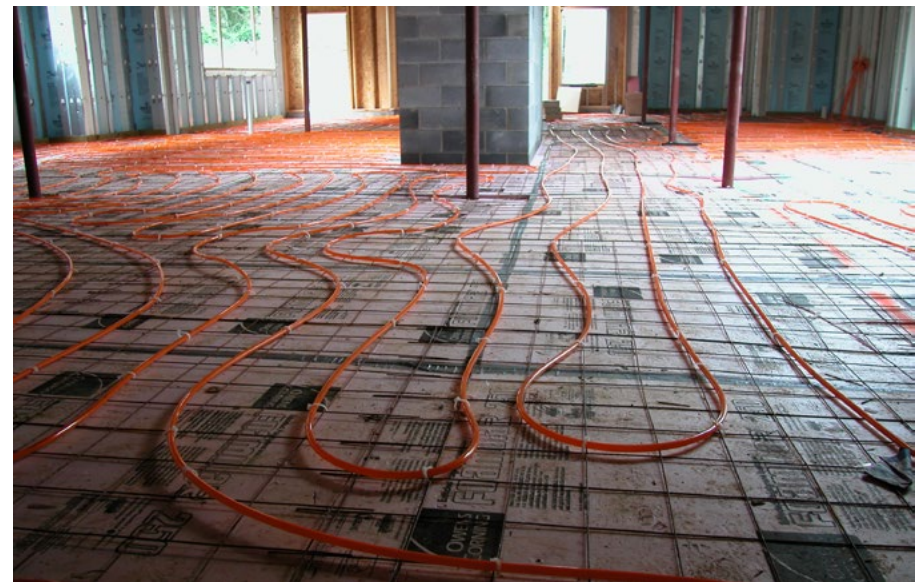
The basement level Watts HEPEX tubing ready to receive concrete overpour.
