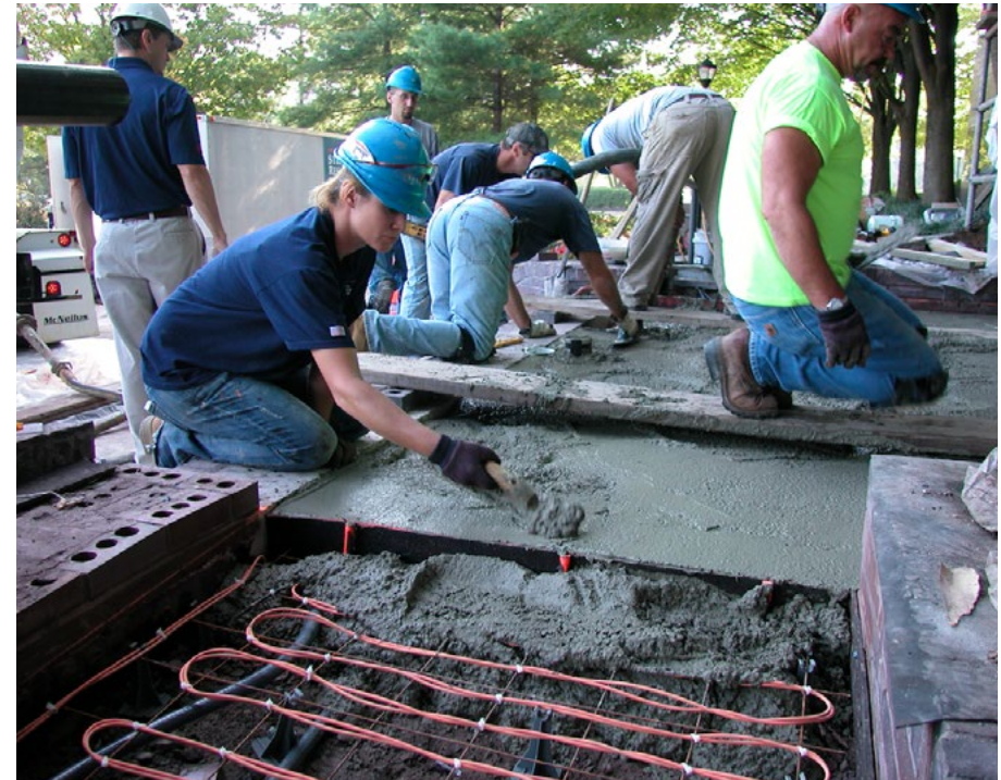
Concrete finishing in progress.
