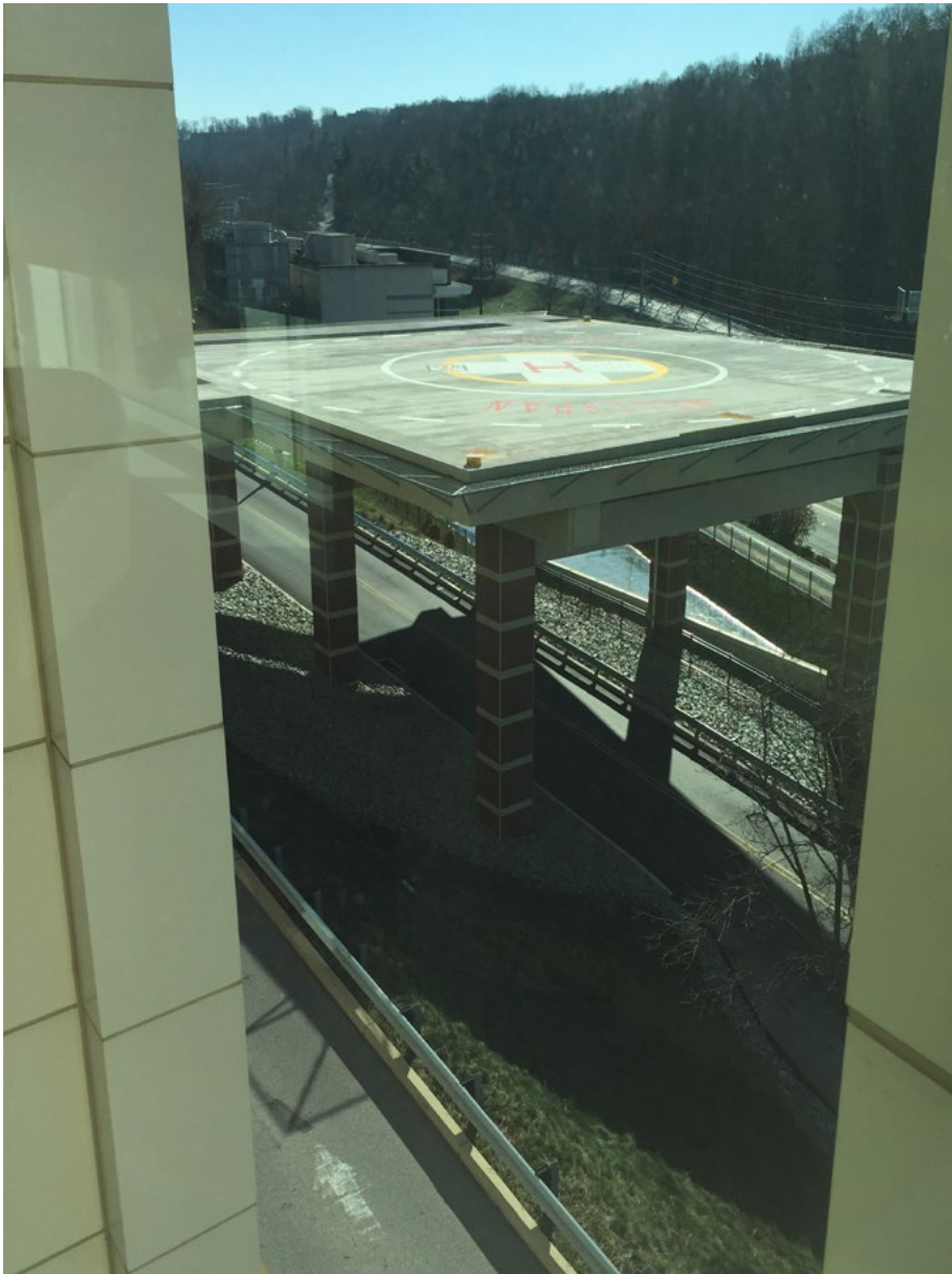
The hospital's new helipad, and other radiant snow melt areas, have been in operation for more than five years.
