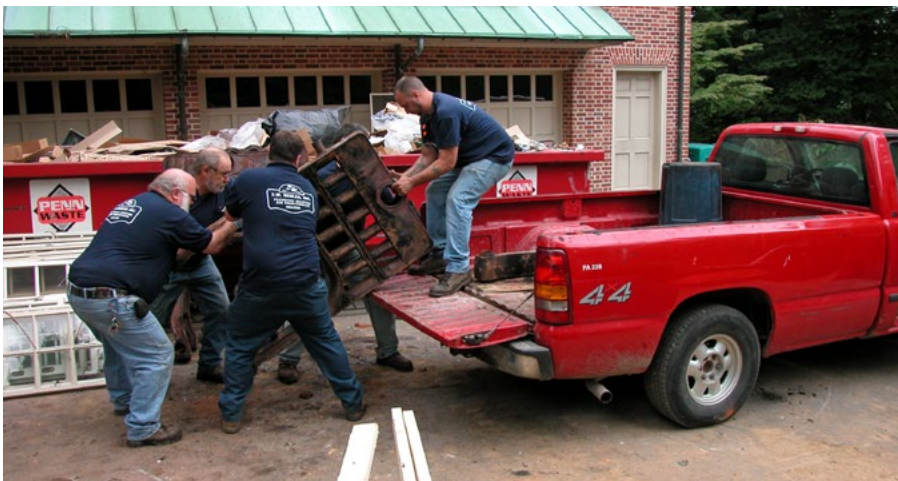
The F.W. Behler crew load a cast iron section to be recycled.
