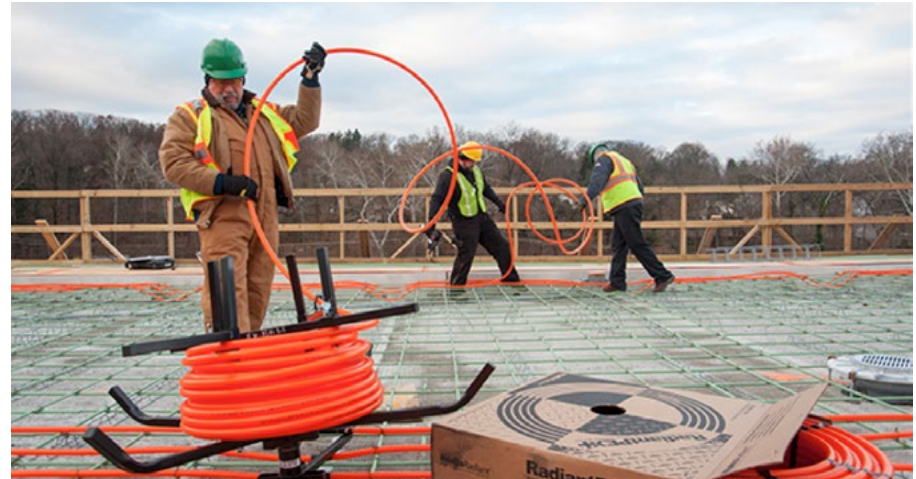
Jeff Ream , the project manager, chose to subcontract the helipad project to our firm.
