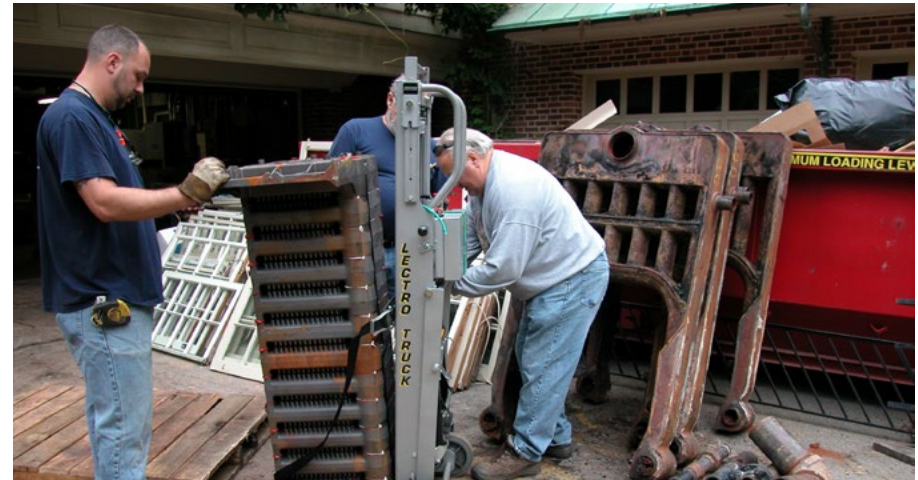
The F.W. Behler crew load a cast iron section to be recycled.
